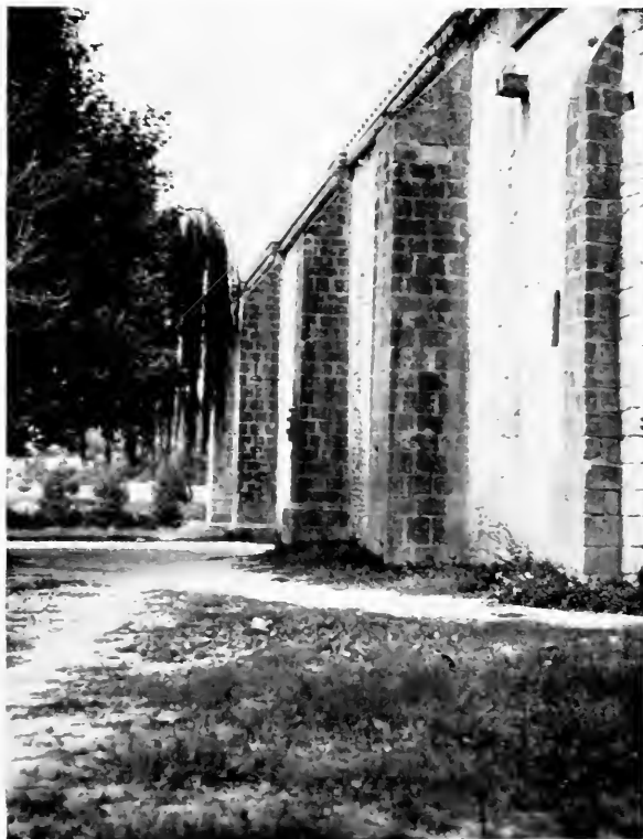
“THE SOUTH WALL WHICH IS CLEARLY SEEN FROM THE ROAD.”—VAISON.
